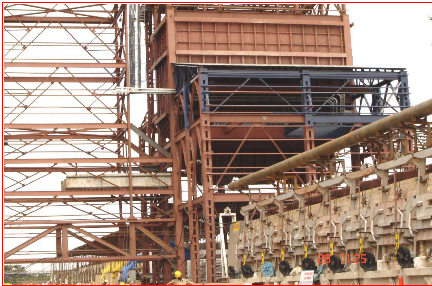
OVENS UNDER INITIAL HEATING
