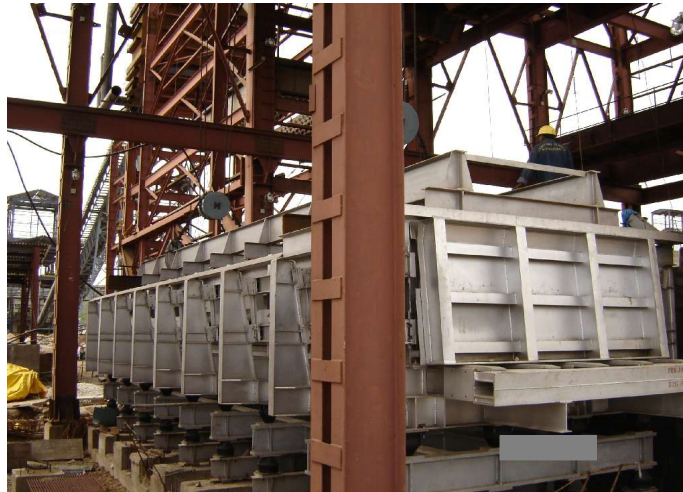
A VIEW OF COMPACTING MACHINE ASSEMBLY IN PROGRESS
