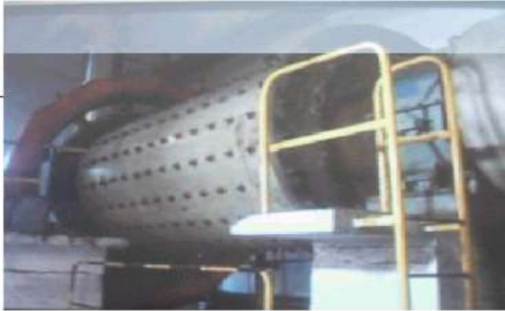
BALL MILL OF THE SESA COKE FINES GRINDING PLANT
